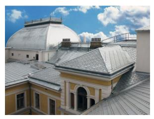
Natural zintek<sup>®</sup> is a bright, even and glossy grey rolled metal. When exposed to the weather, the surface develops a self-protecting layer, which remains stable over time and lends the surface a natural aged look, with a pleasant slate-grey appearance.
